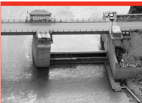
Upgrades are being made to the inlet control structure.
