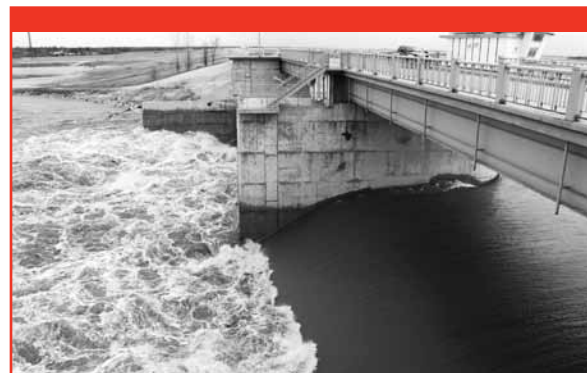
The inlet control structure.
