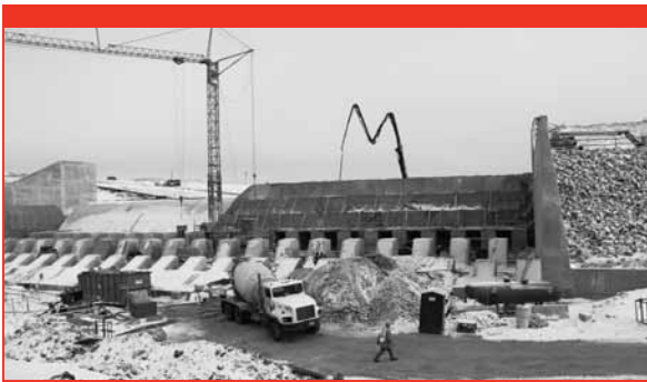
The outlet control structure in Lockport.
